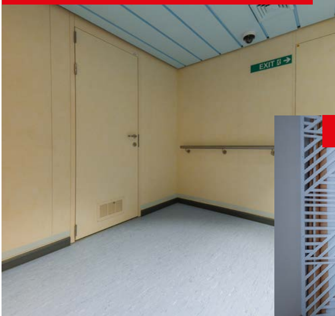
Interior fire door with ventilation, Carnival Jubilee
